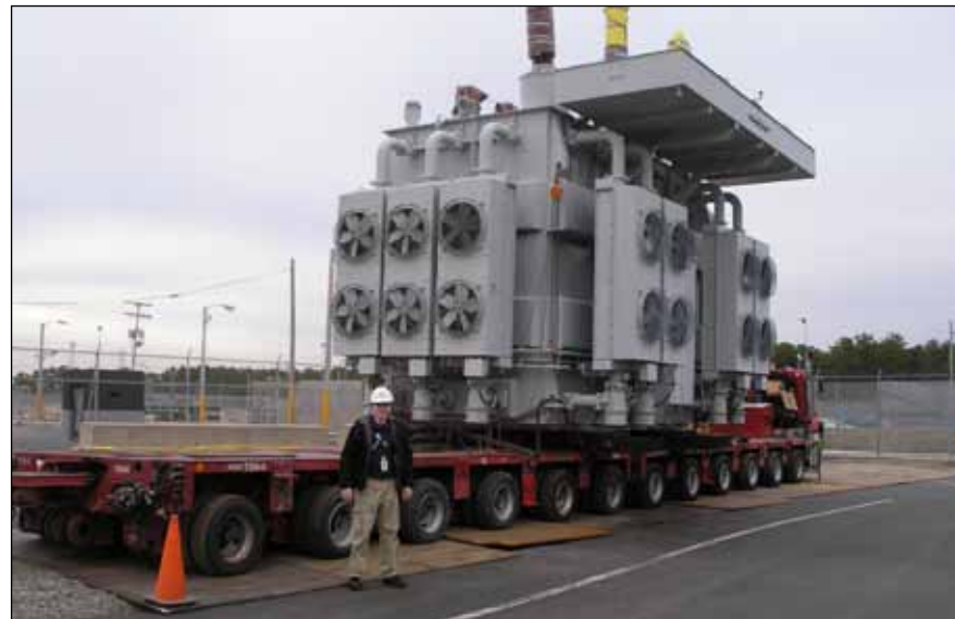
A new transformer being delivered to the Oyster Creek nuclear power plant, in New Jersey, in 2008.
