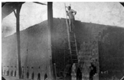
Kilns for burning bricks were massive, Note the openings at the base in which fires were lit to provide the high temperatures needed.
