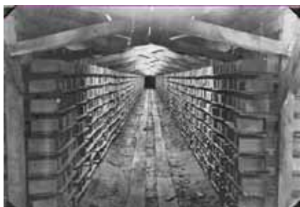
Prior to burning in the kiln, molded bricks were dried on racks in open-sided storage buildings that protected them from damaging rainfall.
