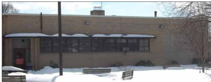
Yorktown Highway Department building exterior.
