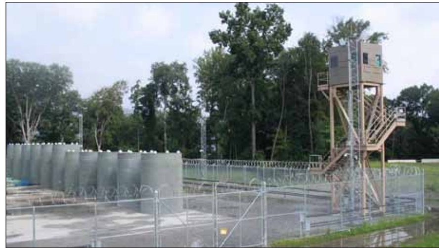
Dry casks stored at Indian Point overlooking the Hudson River in Buchanan, New York.
